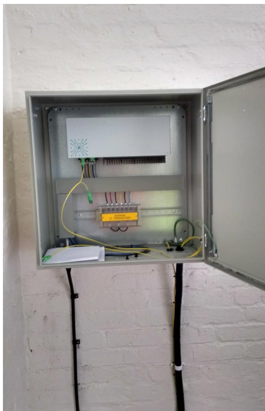
Figure 8: Wall-mounted installation of sensor units at Killin substation
