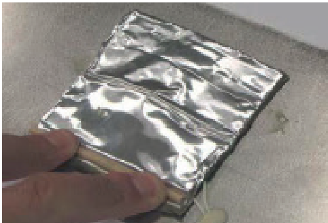
Figure 2.22: Applying and pressing down the covering foil ABM75
