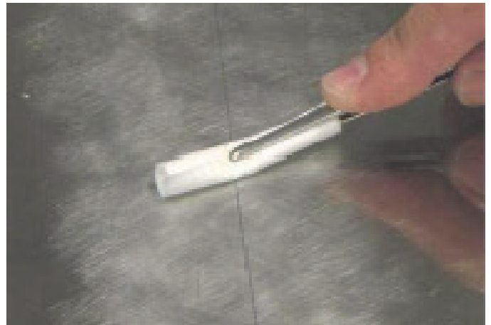
Figure 2.8: Final cleaning of the installation point
